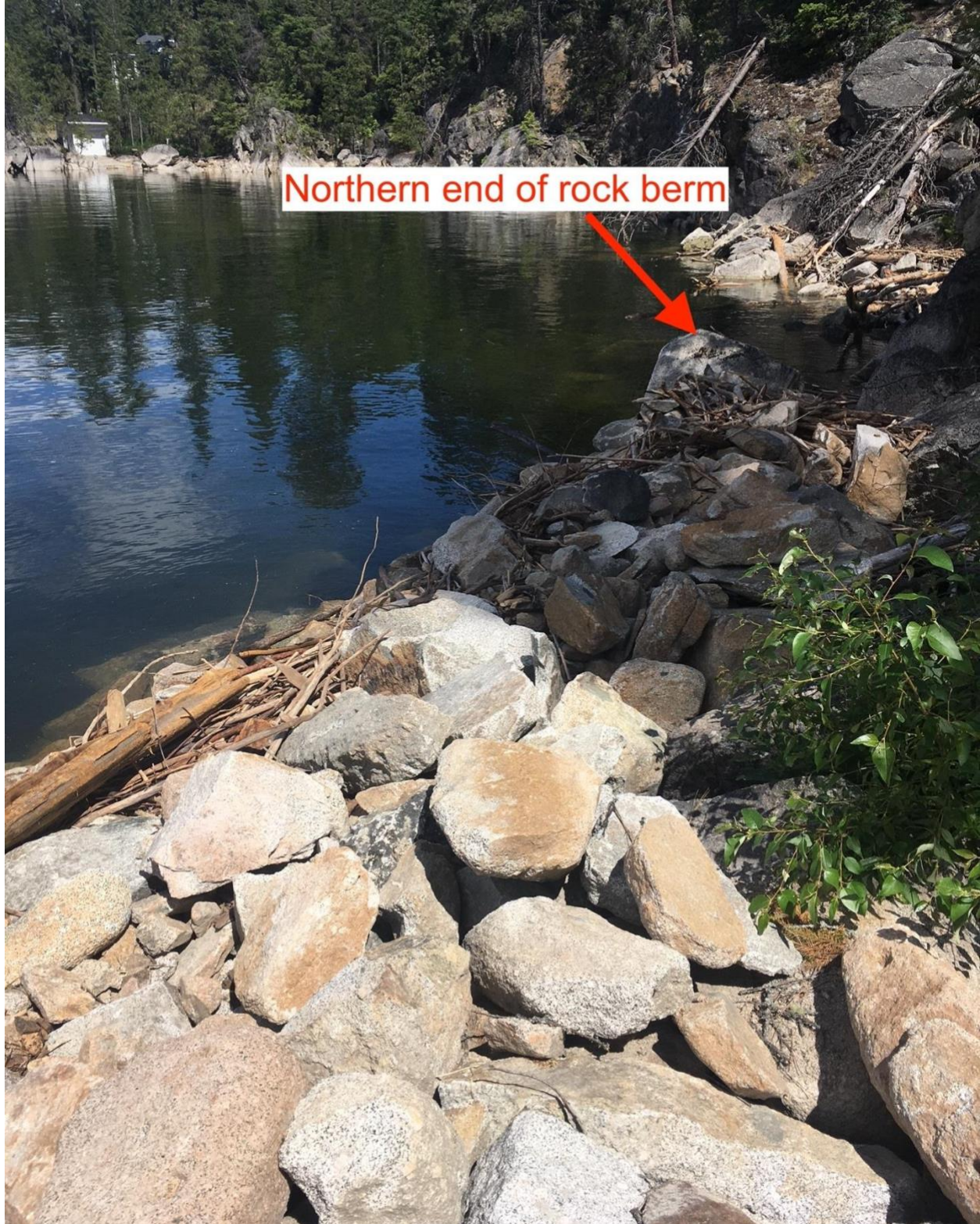
Figure 17. The northern end of the rock berm displaying a collection of woody debris deposited behind during high-water levels.
